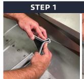
Bend top so that both sides are parallel to metal roof.
