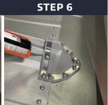
Apply additional sealant around base if desired.
