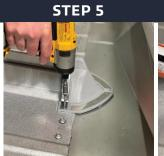
Follow indicated fastening pattern and attach Dek-Cap with fasteners.
