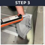
Remove flashing & apply sealant on underside of flexible aluminum edging.
