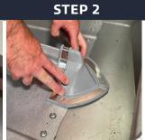
Press Dek-Cap edges into contours of panel configuration.
