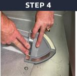
Slide Dek-Cap flashing over panel profile.
