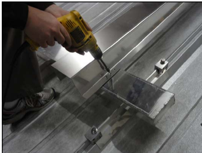
5. Locate Platform Channels to fit equipment to be mounted. Top of Platform Channels should be level. Fasten with 3/4" Tek Screws through holes provided.
