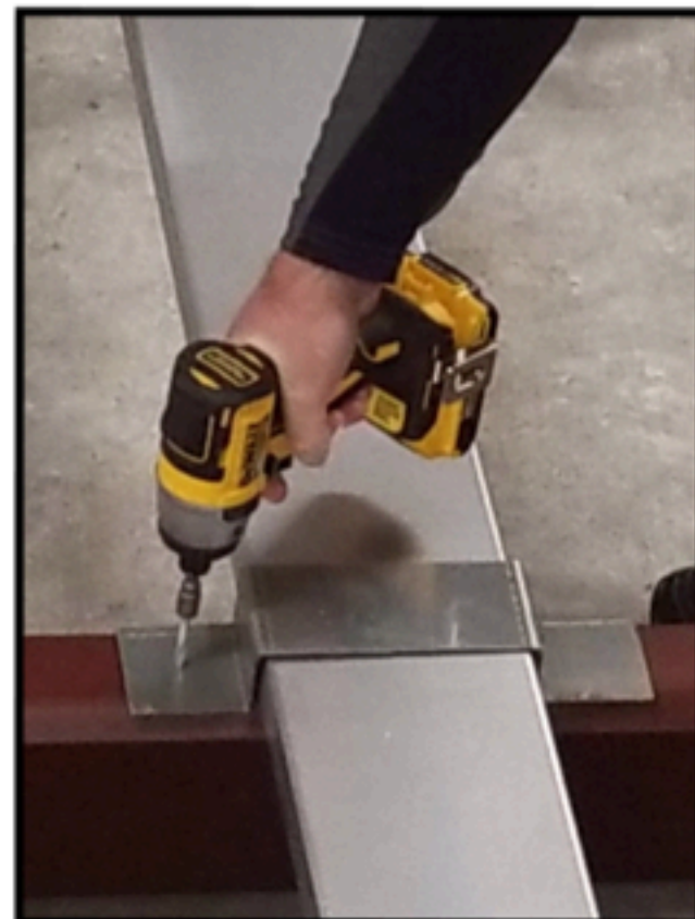
4. Install Hold-Down clips at all four Purlin/Support end conditions. (Hold-Down Clips not required on middle purlin)
