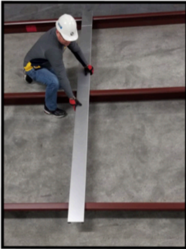
1. Install first side support.
