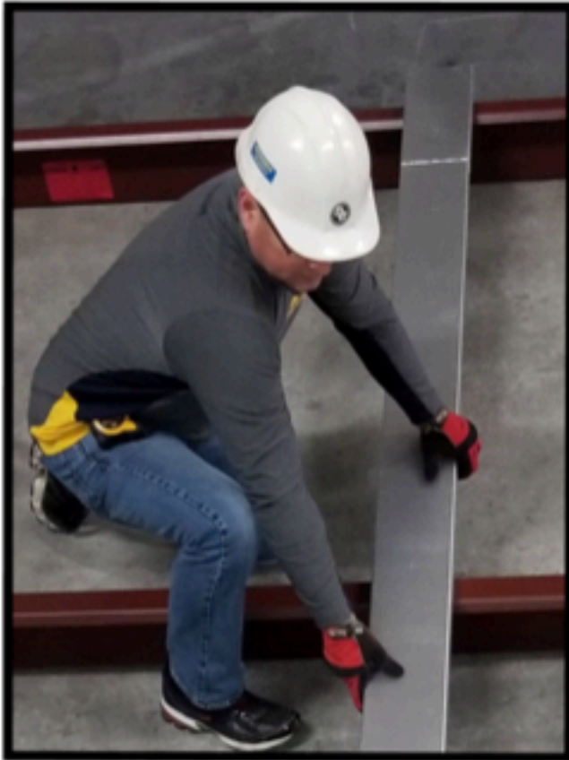
1. Install first side support.
