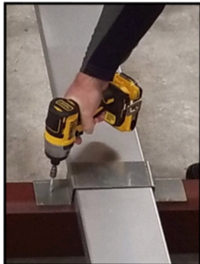
4. Install Hold-Down clips at all four Purlin/Support end conditions.
